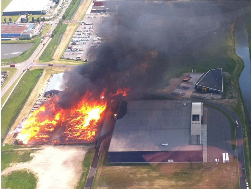
Figure 10 Aerial photo of the fire and the damaged roof on the Asia building (Source: E. Driessen, zelfvliegen.nl)
