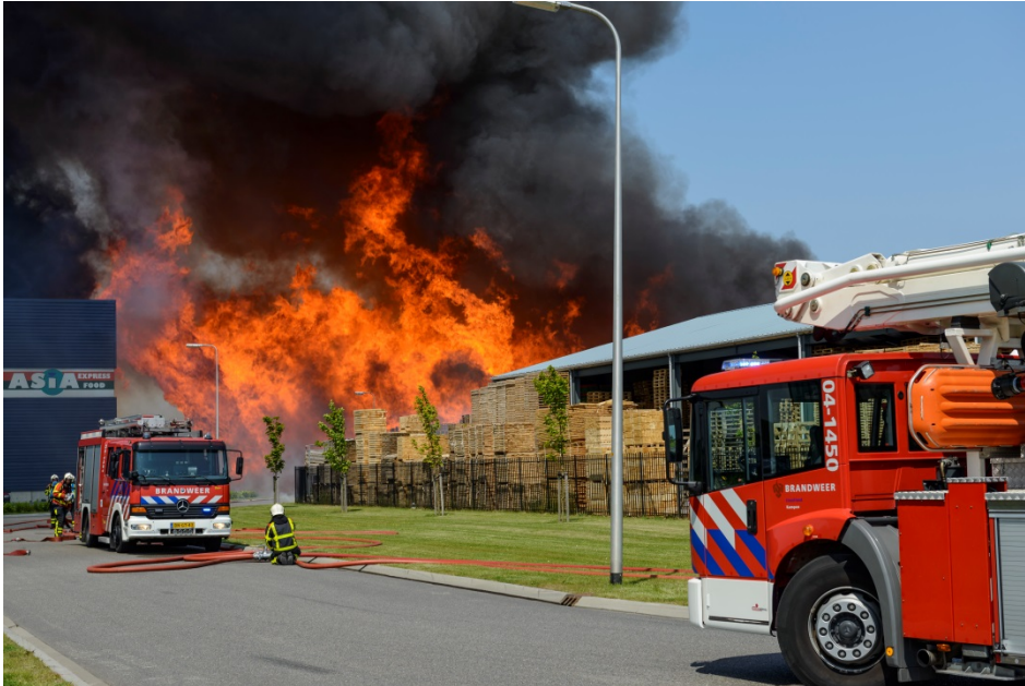
Figure 8 At 13:44h smoke is coming from the roof of the Asia building (Source: Sjoerd van der Wal Fotografie)
